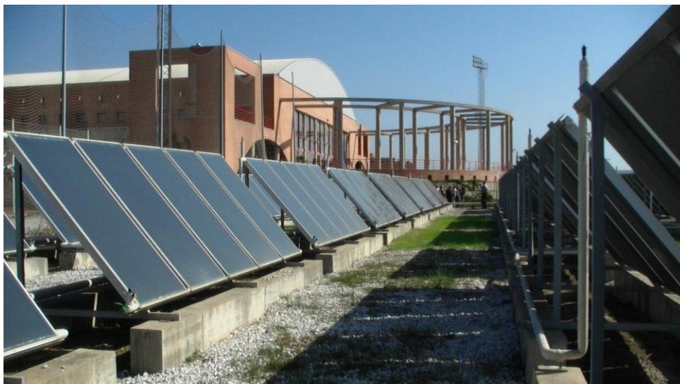
*Flat plate thermal system for water heating deployed in front of the University of Malaga, Spain*
