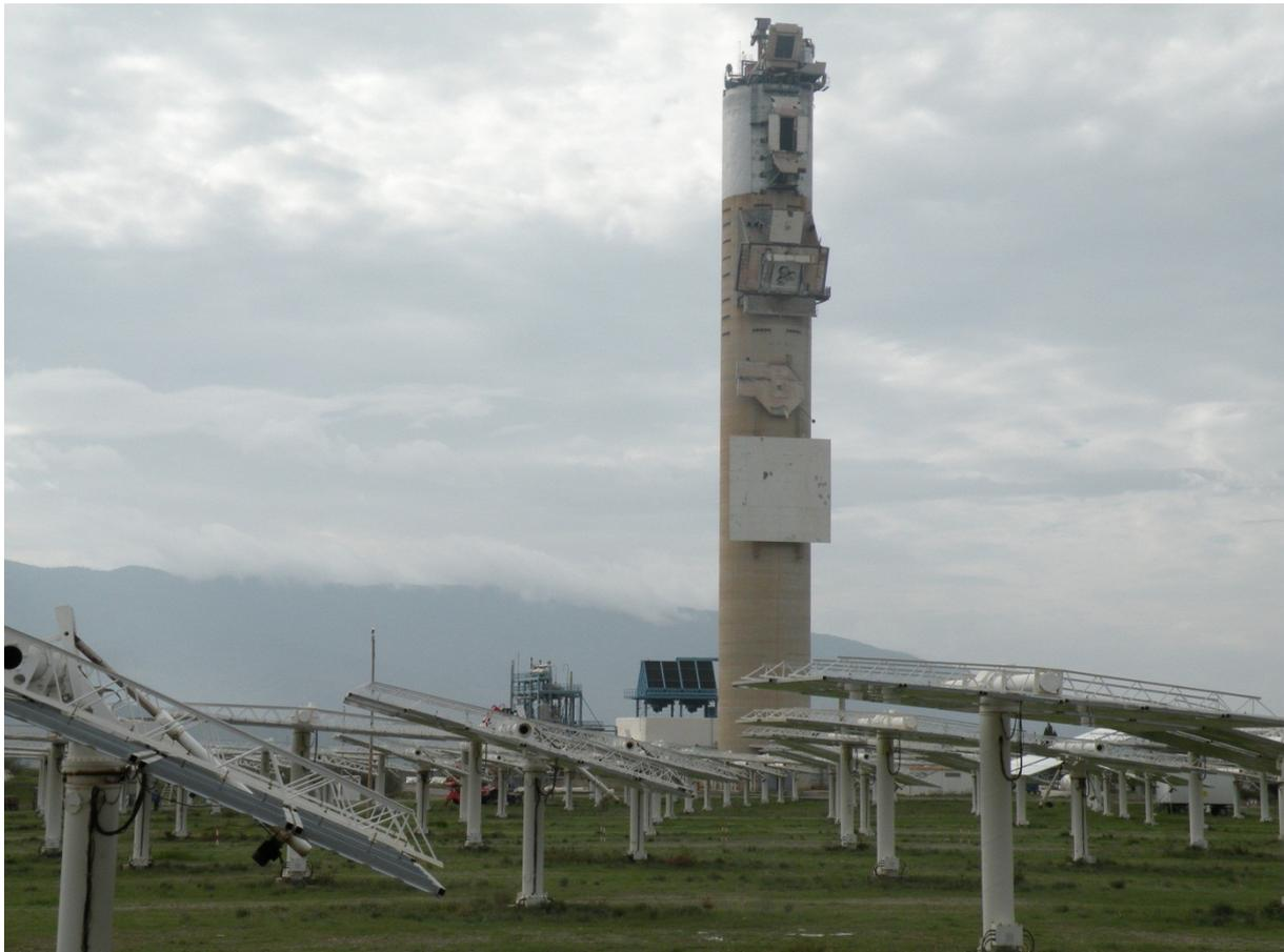
*This is a Solar Tower Power Plant CESA-1, with 300 heliostats with 40 m<sup>2</sup> each, 7 MWth, 83 m height.*
