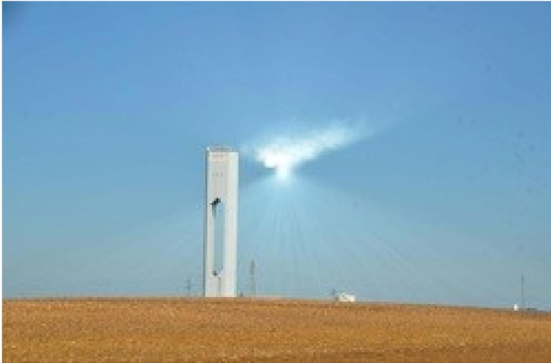
The **PS10 Solar Power Plant** is the world's first commercial concentrating solar power tower operating near Seville in Spain.
